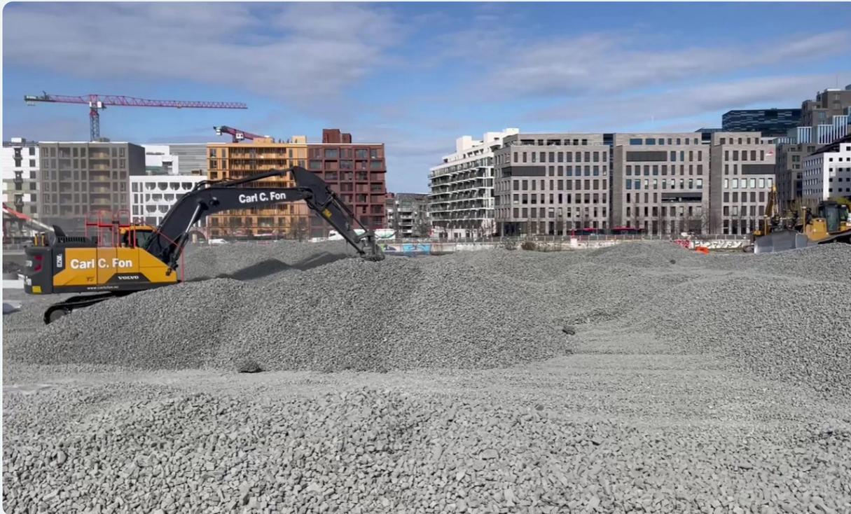
*30 000 cubic metres of Glasopor foam glass aggregate were installed to prepare and level the ground in the park area.*
